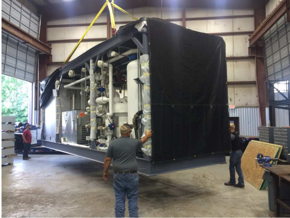
Exhibit 7. Membrane Skid Being Lifted onto the Trailer-truck at the Fabrication Shop.
