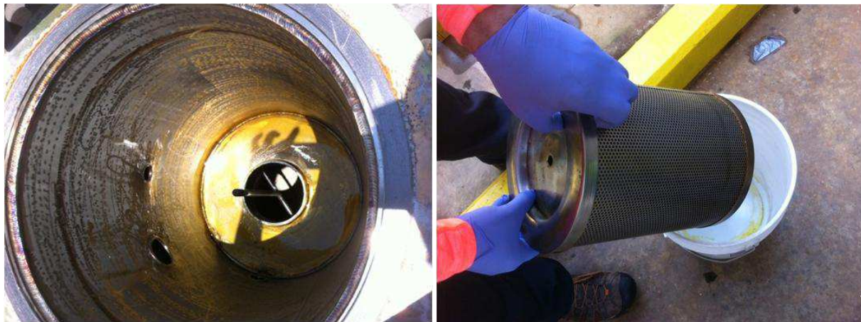
Exhibit 30. Photographs of Compressor Knock-out Vessel (left) and Coalescing Filter Element (right)
