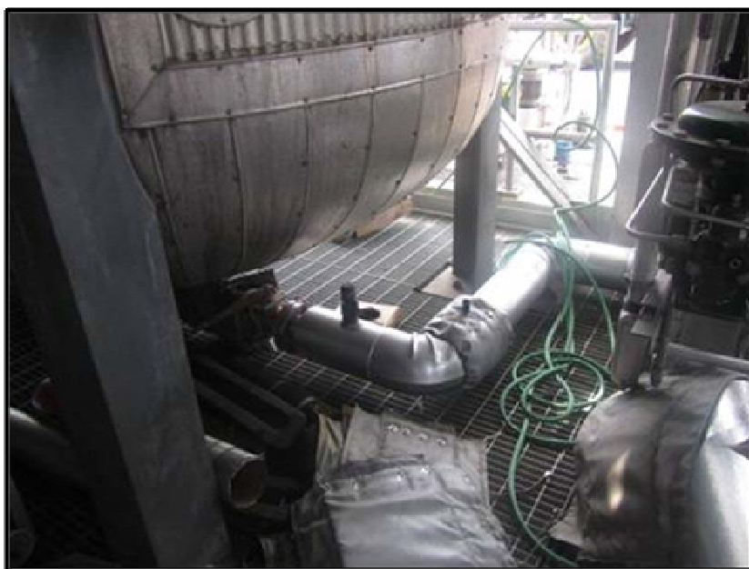
Figure 14: Vessel Drain Header Outlet Connection to TK401
