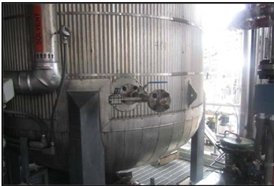
Figure 17: CO 2 Injection Nozzle on TK401
