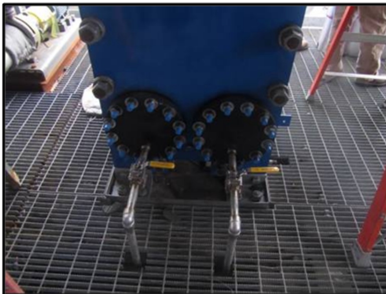
Figure 16: Cross Heat Exchanger Drains
