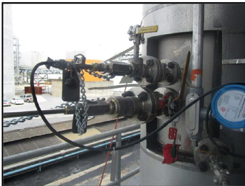
Figure 18: Electrical Resistance Probe (Top) and Retractable Coupon Holder (Bottom)
