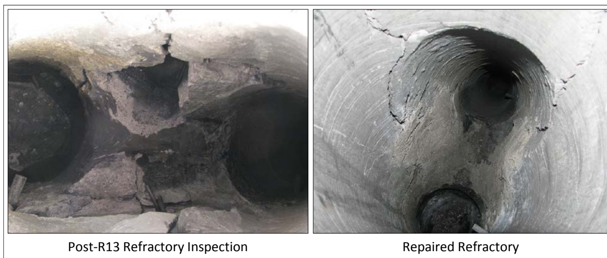
Figure 18. Seal Leg Refractory before and after Repairs
