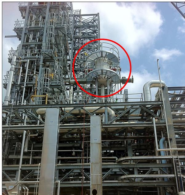
**Figure 3. GE Global Desorber Unit Installed in PSTU Structure**
