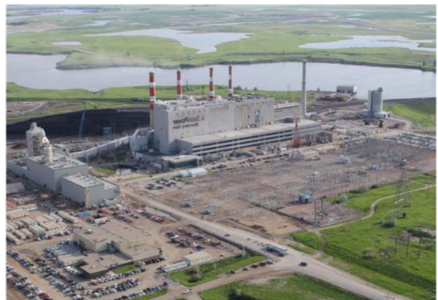
Figure 8: Completed Capture Plant Integrated with Power Plant
