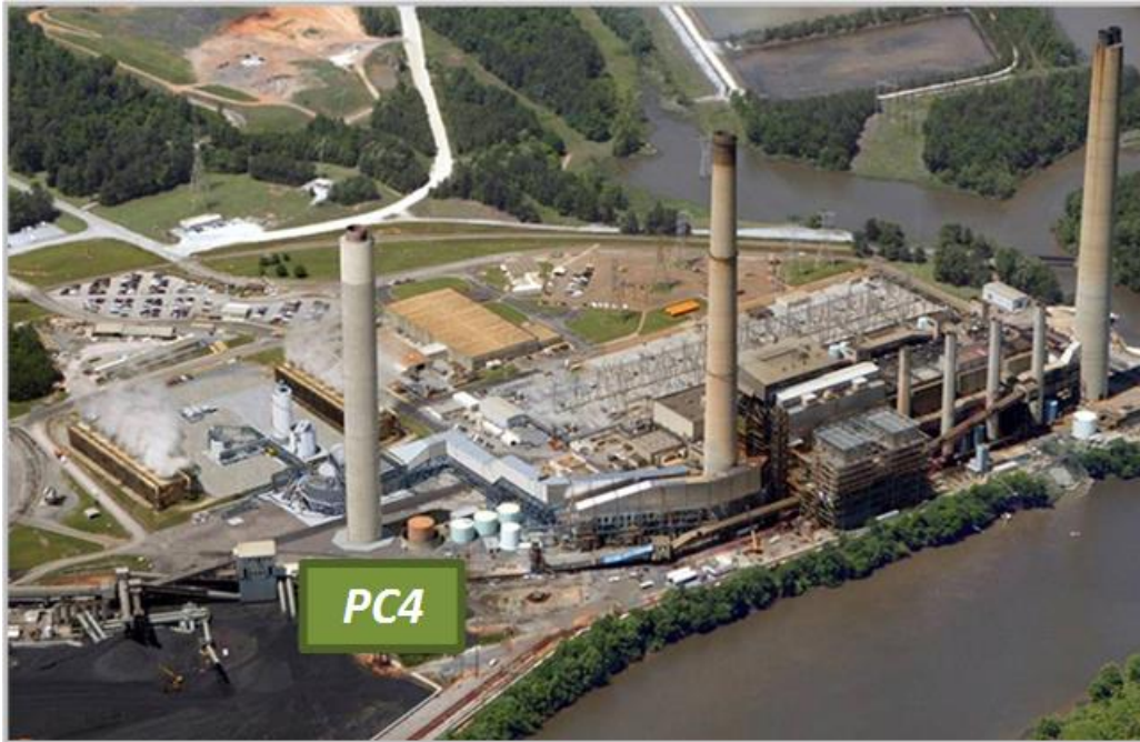
Figure 3. Alabama Power Gaston Steam Plant with PC4 Location
