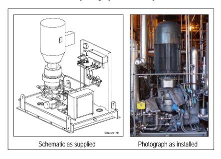
Figure 7-2. Schematic and Photograph of Recycle Gas Compressor.
