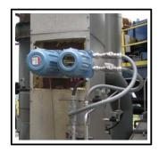
Figure 2-7. Dual O<sub>2</sub>/CO Analyzers.
