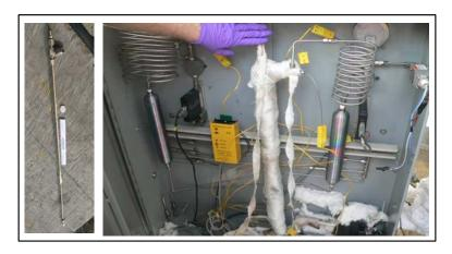
Figure 5-9. MPT Carbon Molecular Sieve Membrane Installed at PSDF.
