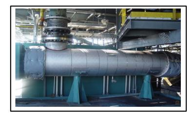
Figure 2-5. Coal Mill Electric Heater.
