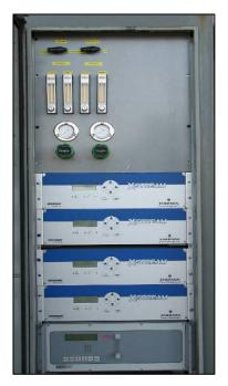
Figure 6-22. Continuous Analyzer Cabinet for PCD Inlet Gas Analysis.
