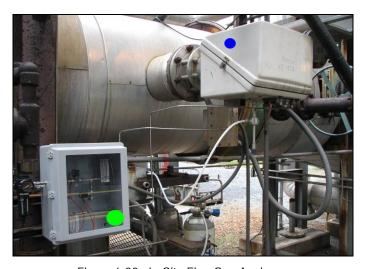
Figure 6-23. In-Situ Flue Gas Analyzer.
