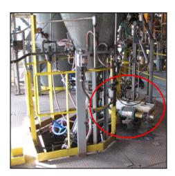
Figure 6-13. Solids Sample System at Coal Feeder Surge Bin.
