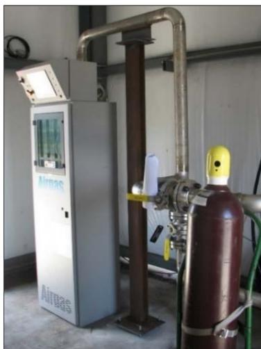
Figure 10. Nitrogen Dioxide Gas Containment and Delivery Cabinet
