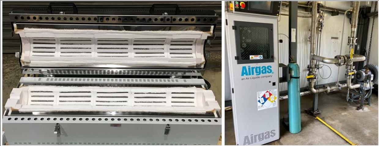
**Figure 11. Sulfur Trioxide Additive System**
